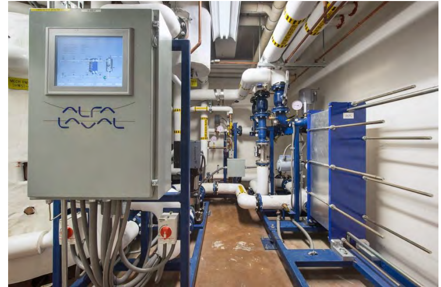
Florence Moore Student Resident Hall Parallel Installation
